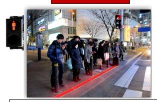
Corresponding with stop signal of existing signal system, switching on the red light means attention.
