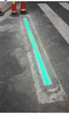
②The embedded parts are put into the cement groove. If the slot space is too large, the two sides of the embedded parts are smoothed with cement paste appropriately.
