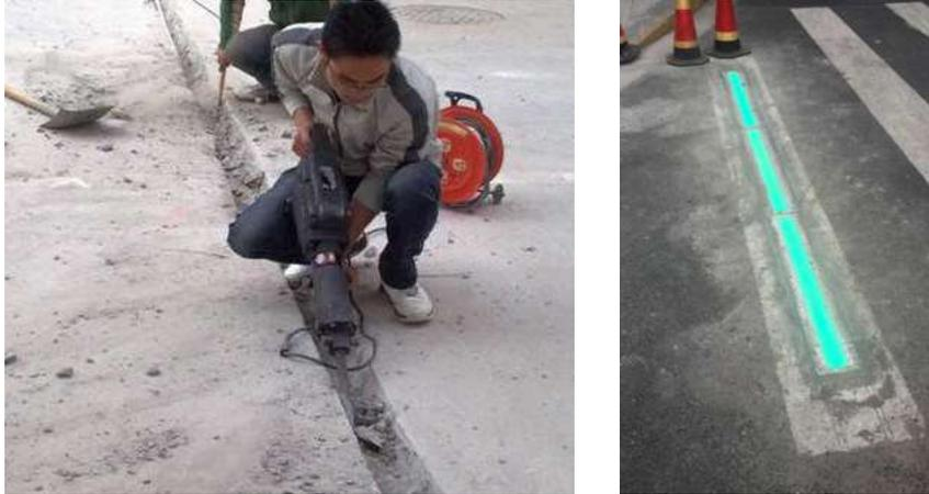
② The embedded parts are put into the cement groove. If the slot space is too large, the two sides of the embedded parts are smoothed with cement paste appropriately.
